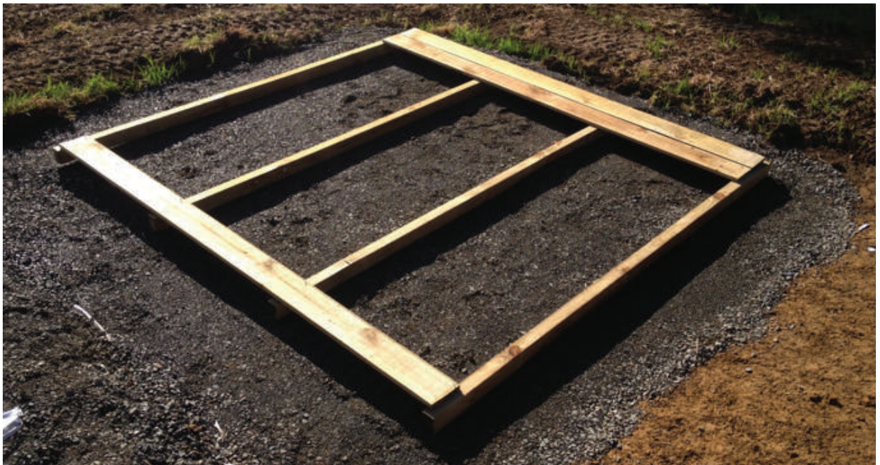
Four bearers with the first three floor boards.
